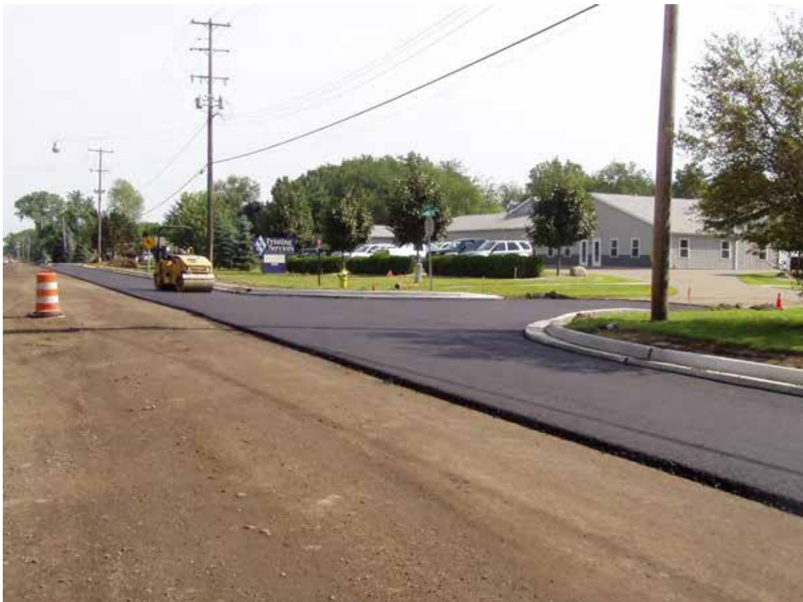
S. Sprinkle Road Base Course Paving – Pavilion Township
